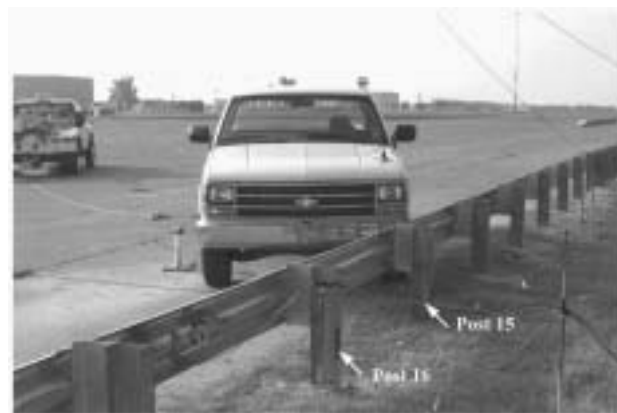
Figure 1. A picture of the G4(1S) system before crash test 405421-2.
